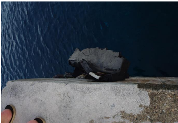
Damaged Fender - Jaluit
